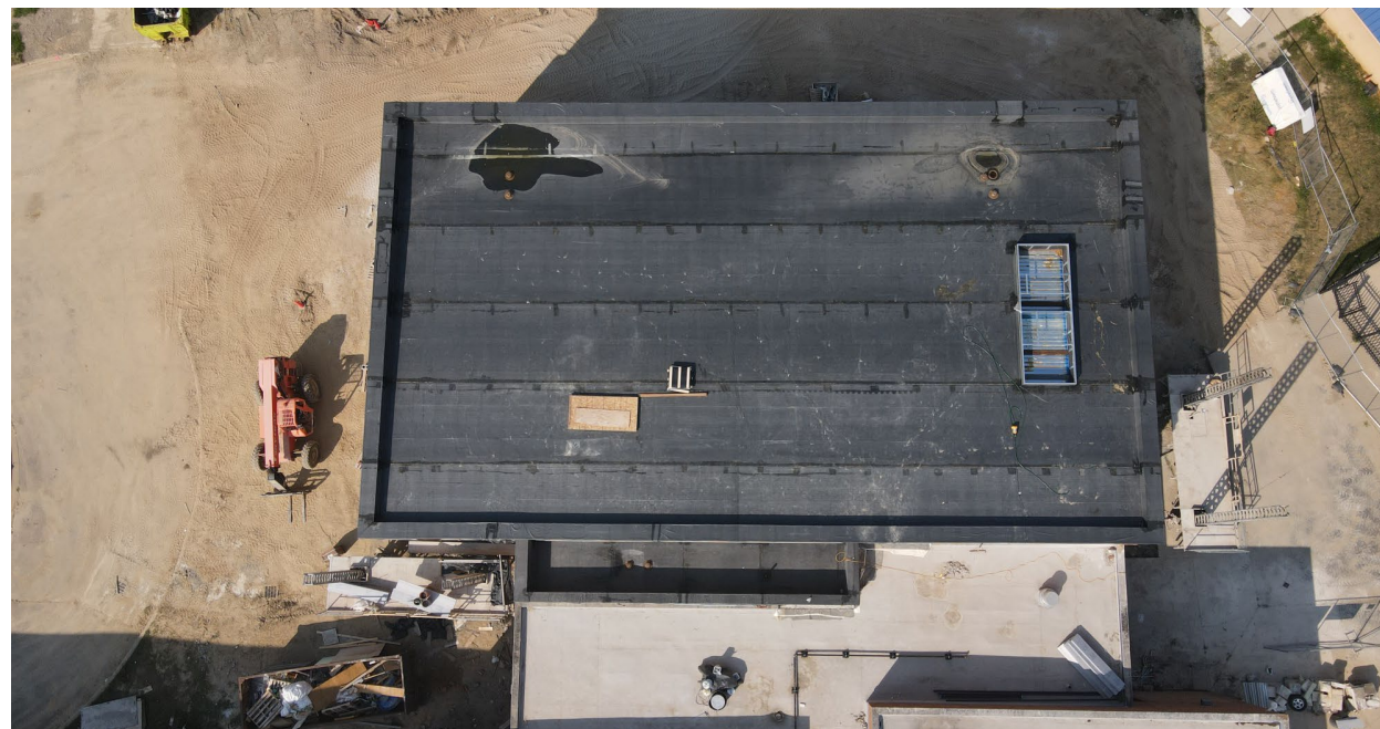
Farmington HS – New Addition Roofing
