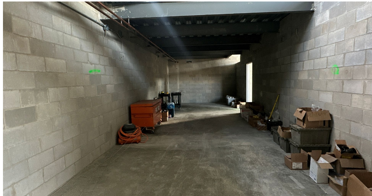
Farmington HS – Storage Room
