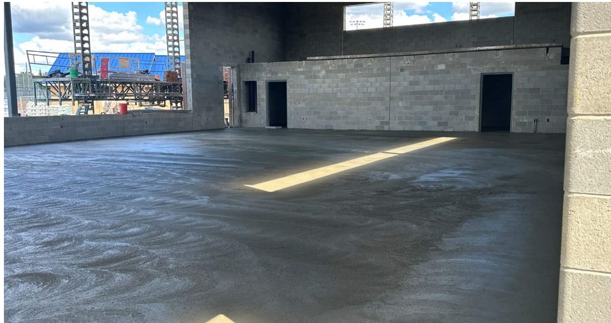
Farmington HS – Interior Looking East
