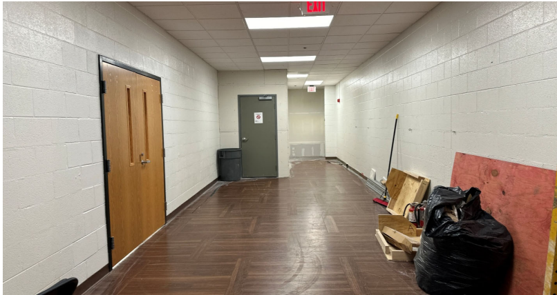
Farmington HS – Interior Corridor
