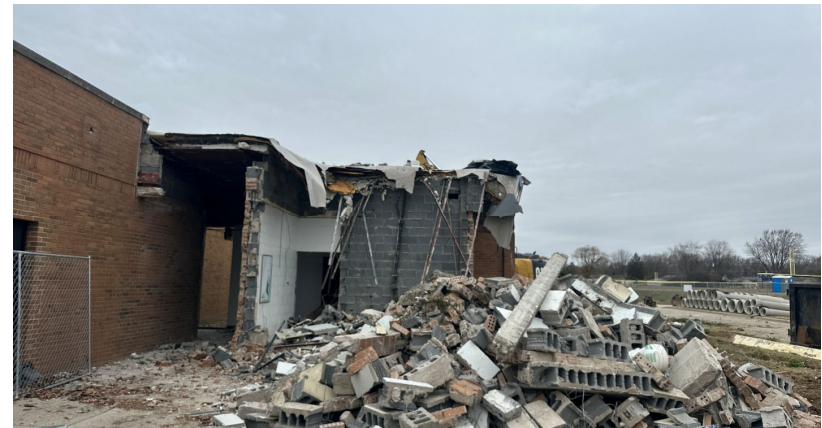
Farmington HS – Demolition
