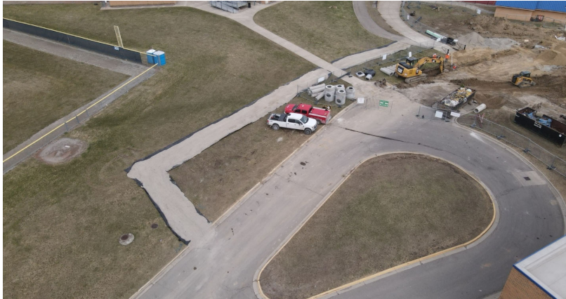
Farmington HS – Temporary Pathways
