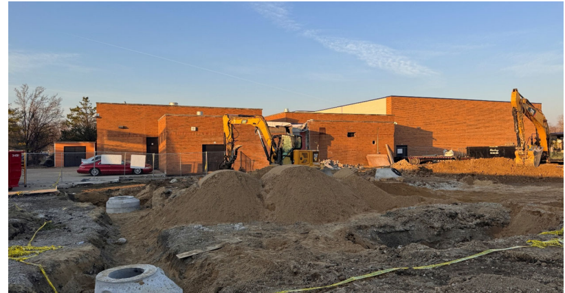
Farmington HS – Site Utilities
