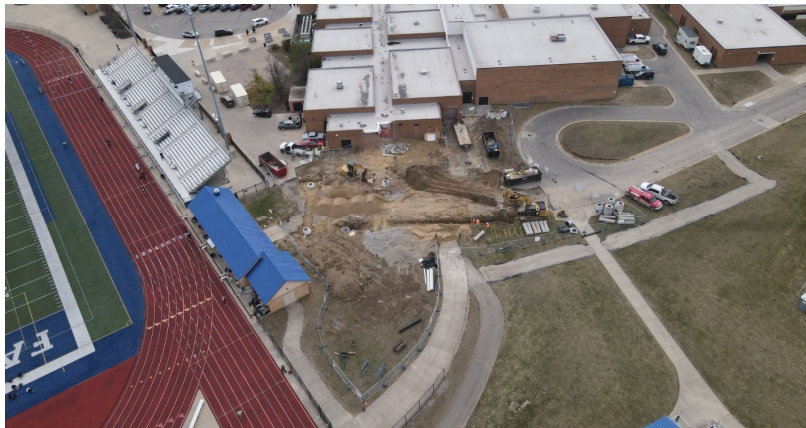
Farmington HS – Demolition
