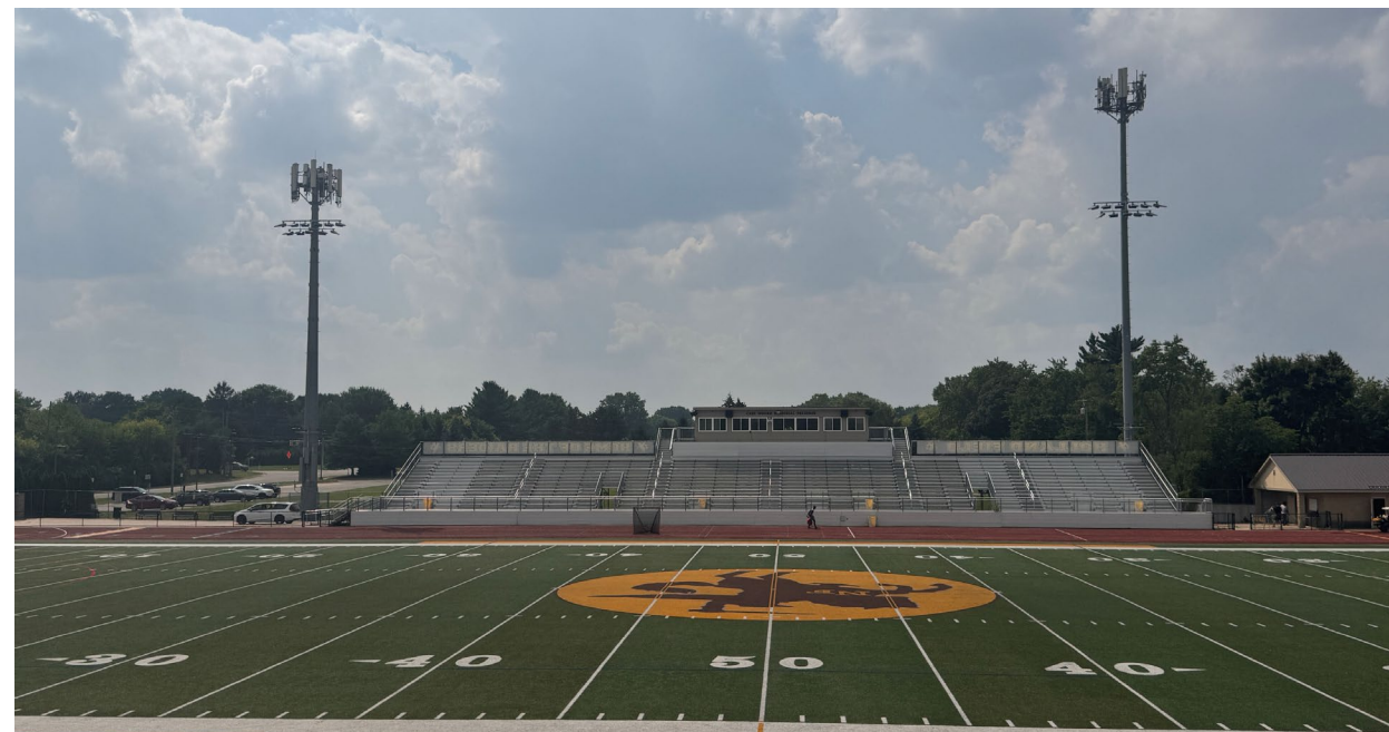
North Farmington HS – Main Field Stadium Lighting
