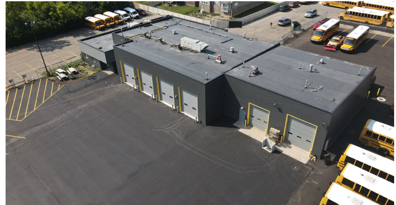
Transportation – Roofing & Service Bay Addition
