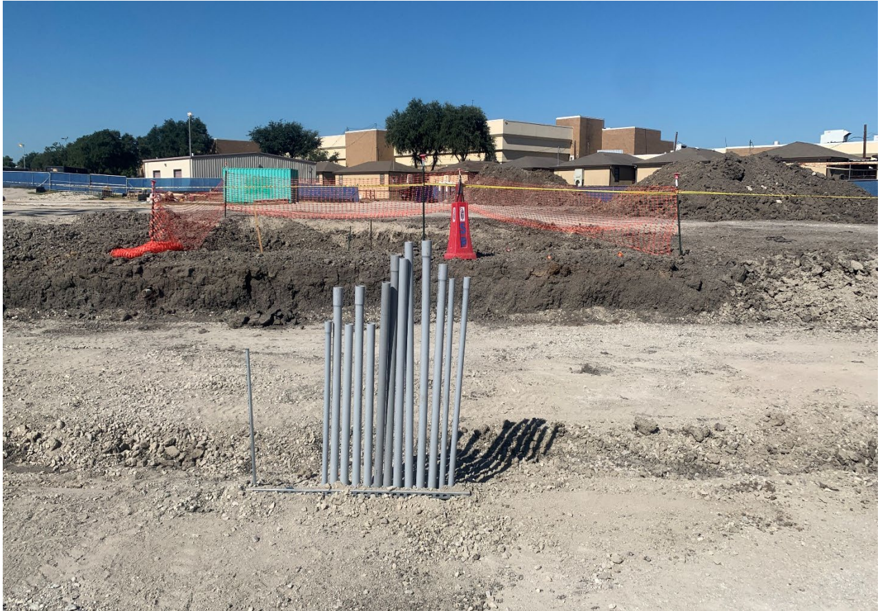
Lakeview HS – Underground Electrical
