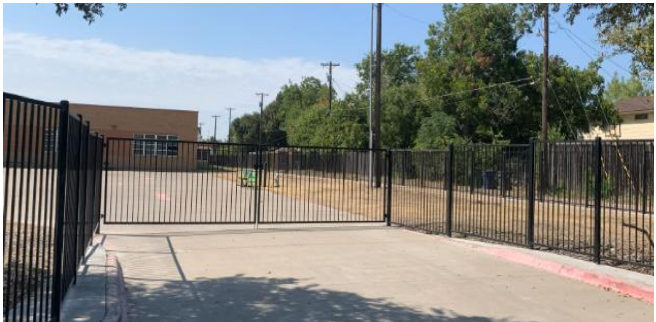
Secure drive gate at Beaver Technology Center for Math & Science
