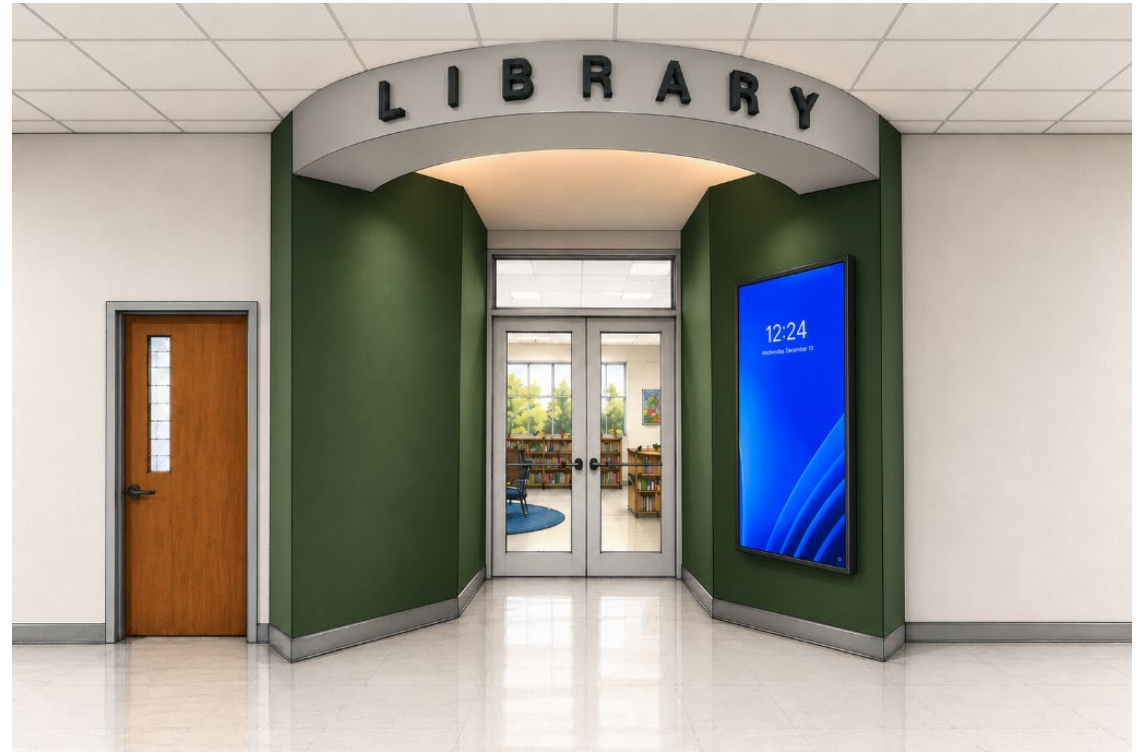
After - Contemporary soffit with aluminum storefront entrance
