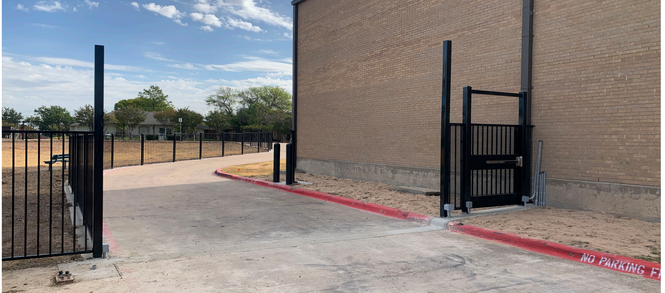
Club Hill Elementary School – Delivery Area
