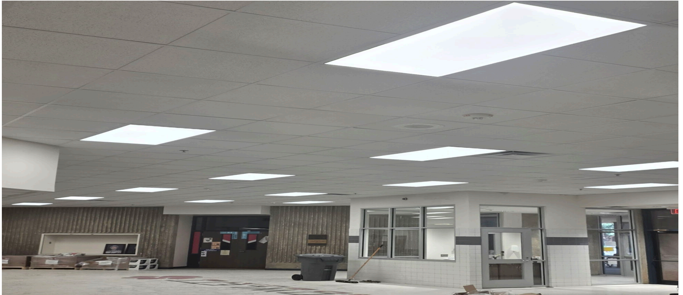
Rowlett Skylights Removed
