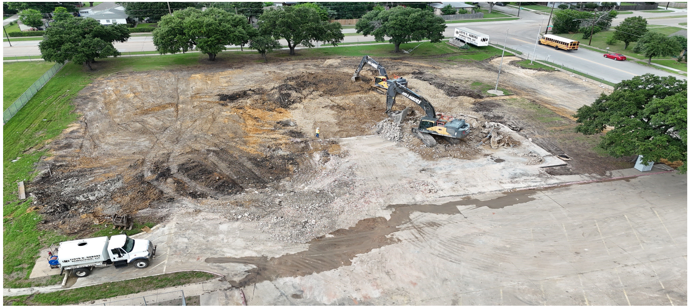
Manuel and Maria Valle Student Services Center Demolition
