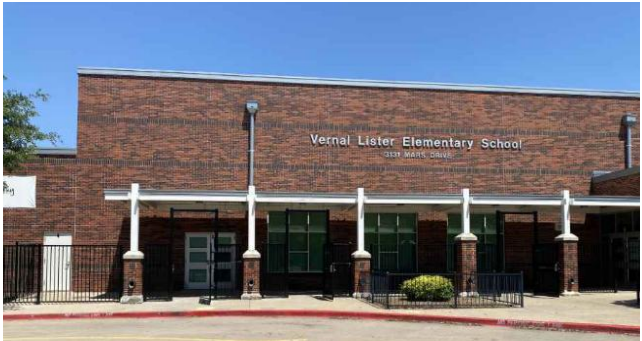
Fence and pedestrian gates at Lister ES.
