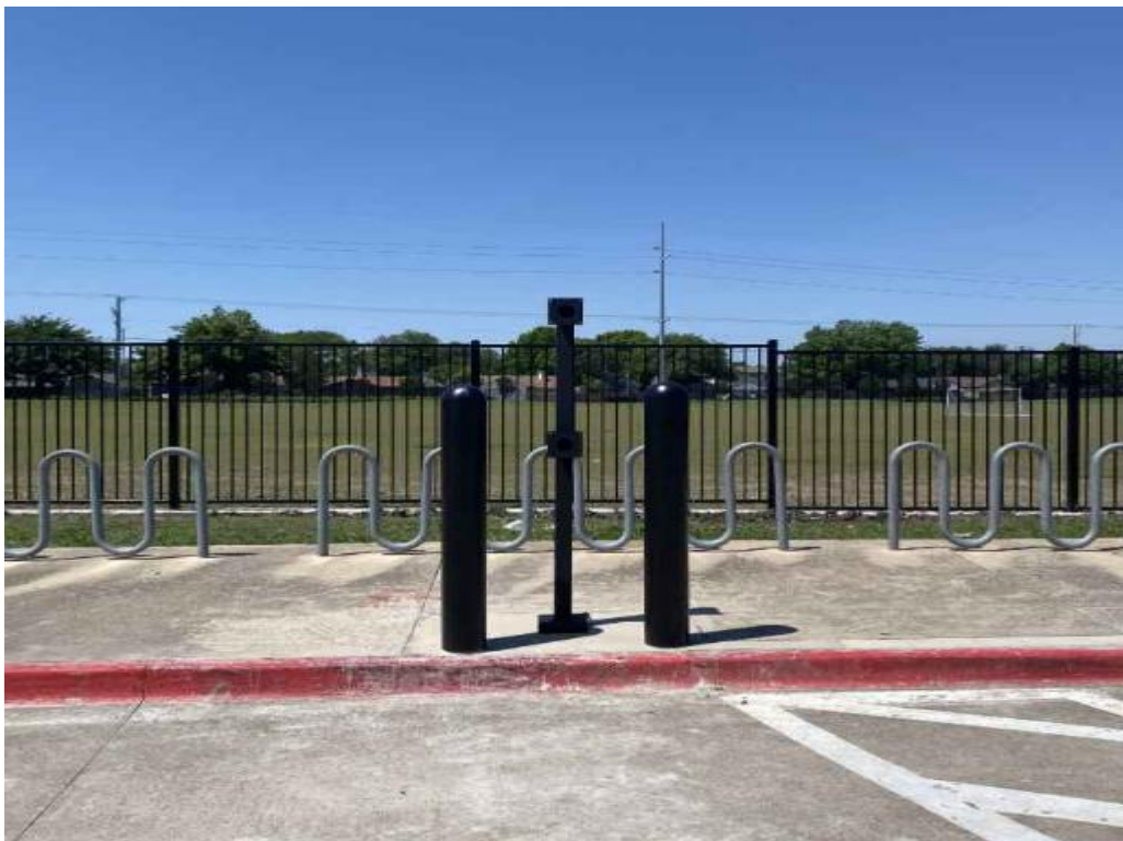
Vehicle Gate Pedestal at Lister ES.
