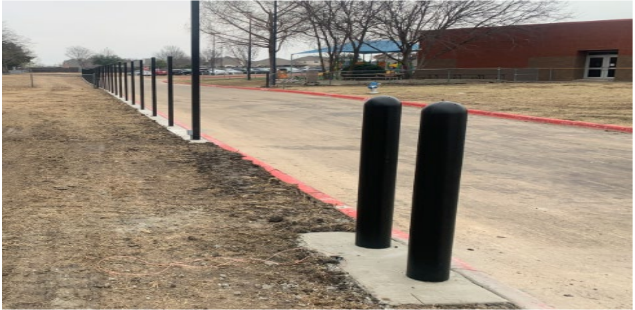
Fence posts, gate bollards and mow strip at Armstrong.
