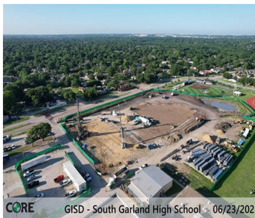
South Garland: Progress
