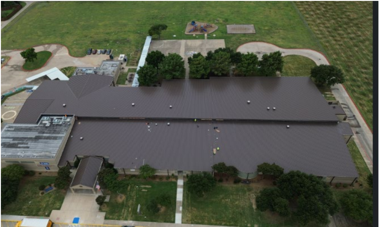
At Herfurth ES, the new gable over the cafeteria will help divert water away from sensitive areas.
