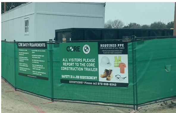
Naaman Forest: Demolition
