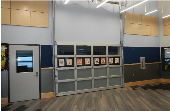
Figure 44 Roll up door to expand classroom
