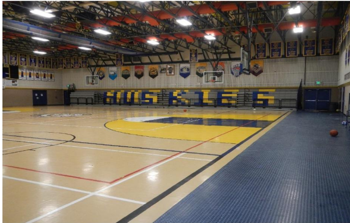
Figure 26 The gym floor sustained some damage from cots when housing displaced residents during the typhoon
