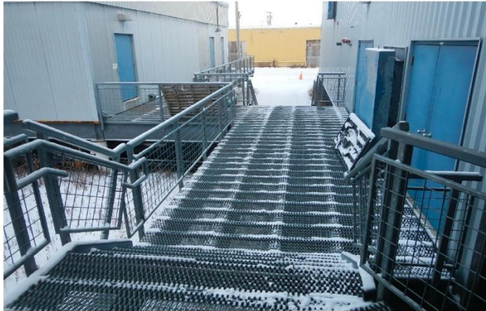
Figure 8 Boiler room and E-generator room on right
