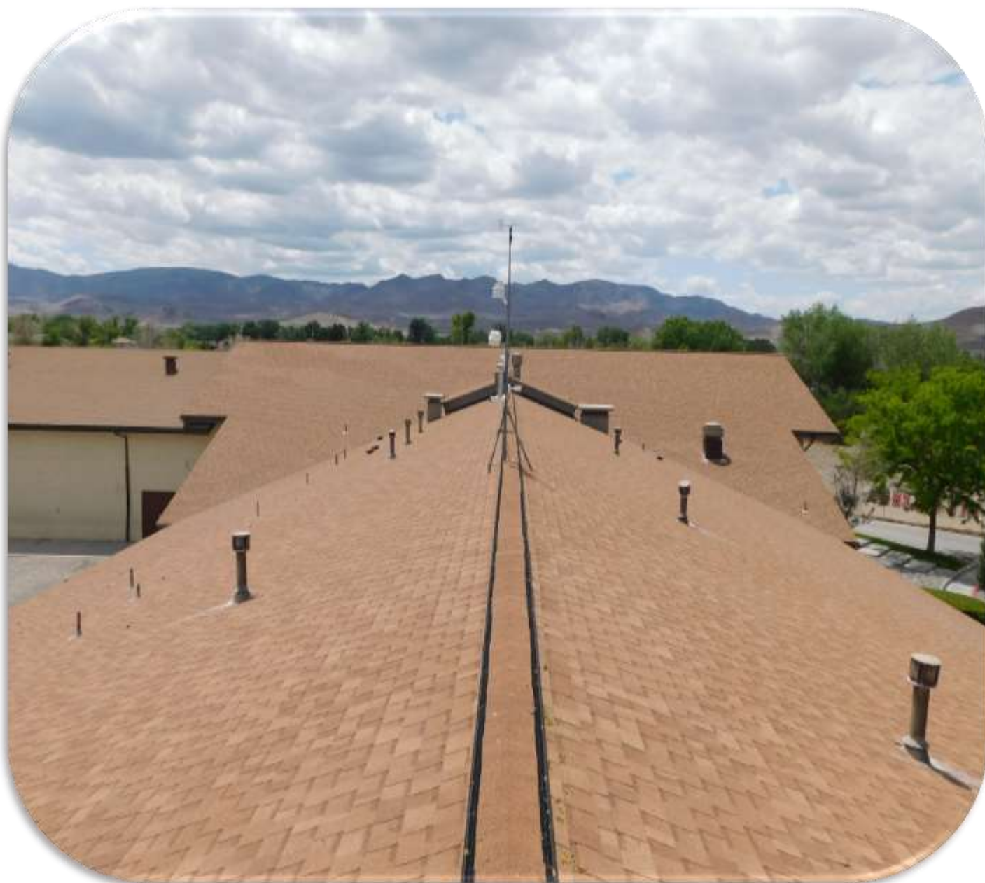
OVERVIEW OF THE MAIN ROOF LOOKING TO THE WEST, STANDING AT THE EAST END.
