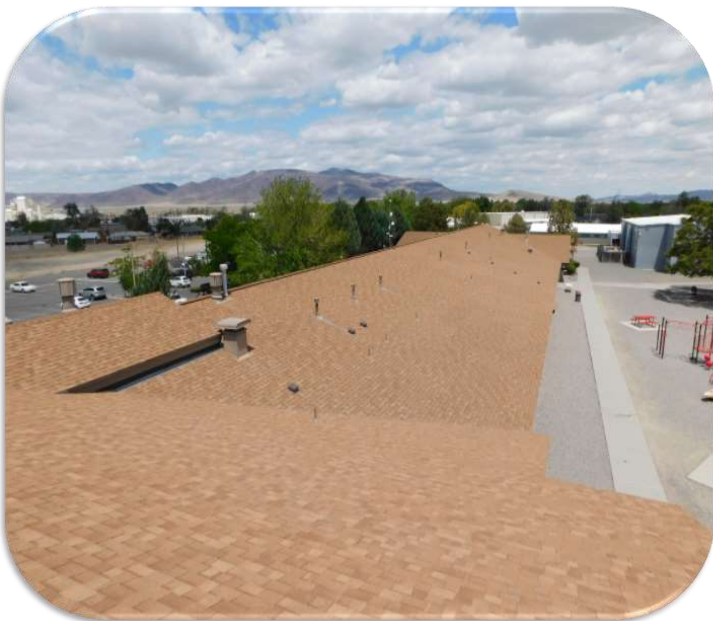
OVERVIEW OF THE MAIN ROOF LOOKING TO THE EAST END.
