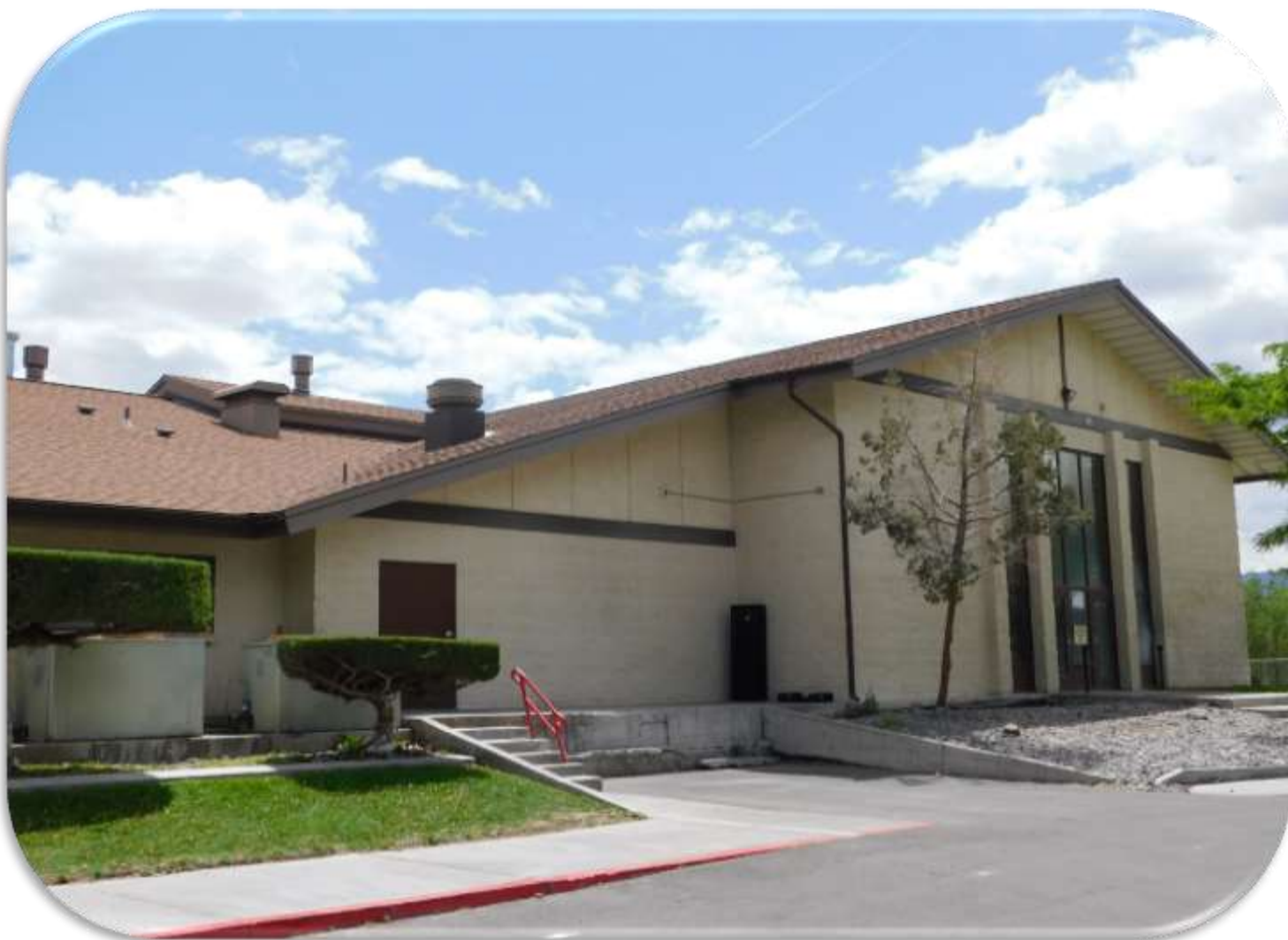
(FIS) STREET VIEW OF THE BUILDING TO BE RE-ROOFED.
