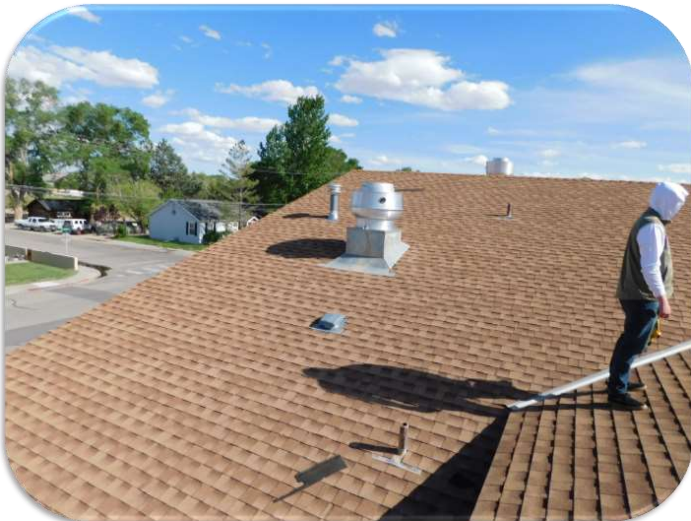
OVERVIEW OF THE NORTH SIDE OF THE MPR ROOF YERINGTON.
