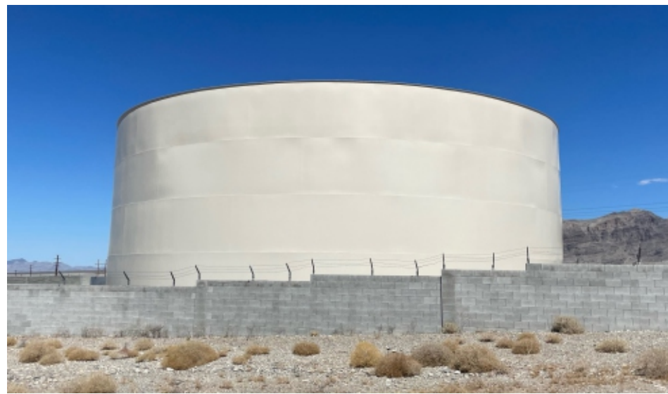
EXISTING (NEWLY PAINTED)
