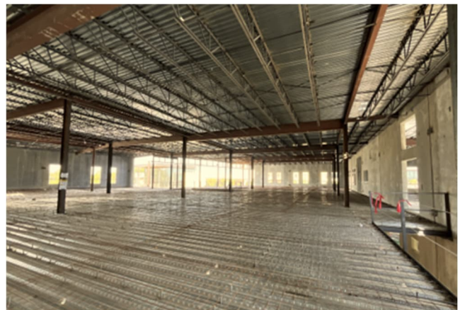
2nd Level Floor Deck
