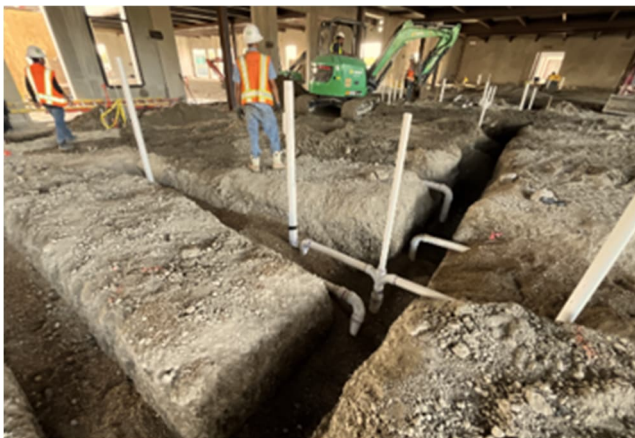
Interior 1st Level Underground Plumbing
