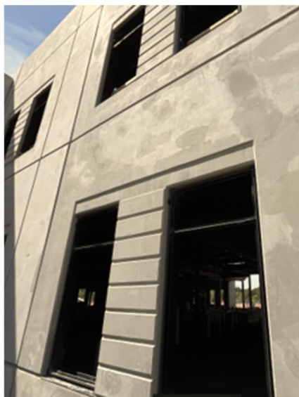
1st and 2nd Level Windows
