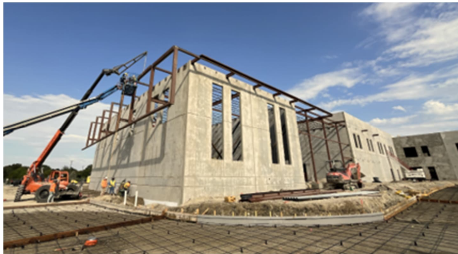
East Side Exterior Steel Framing
