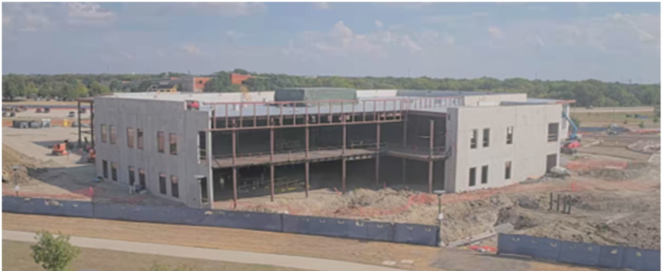
Exterior Steel Framing and Roofing Materials Staged on the Roof
