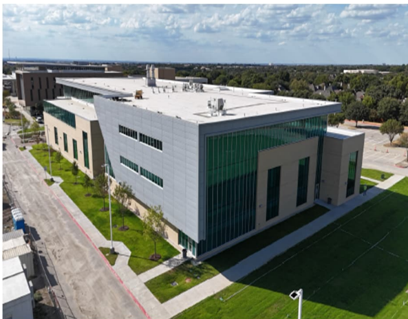
Southeast Corner of Building
