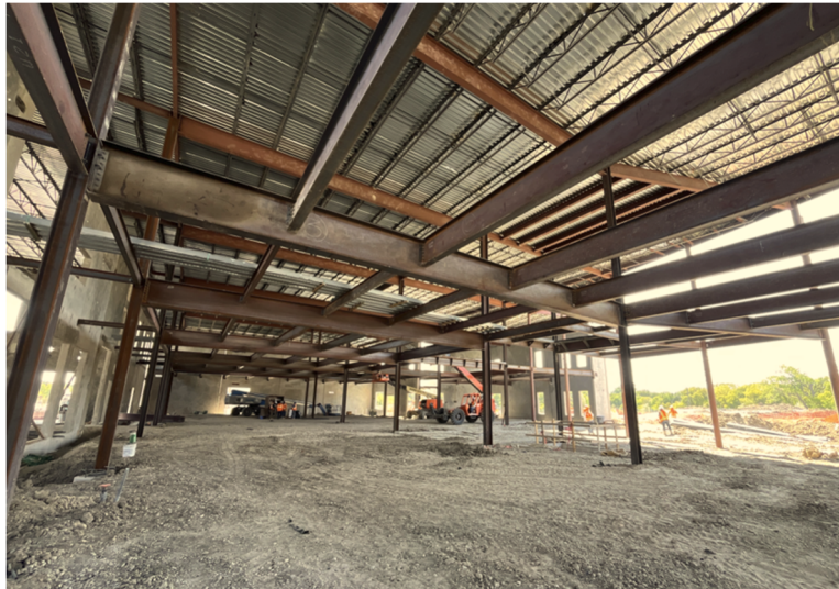
Interior Steel, Framing and Bottom of Roof Deck
