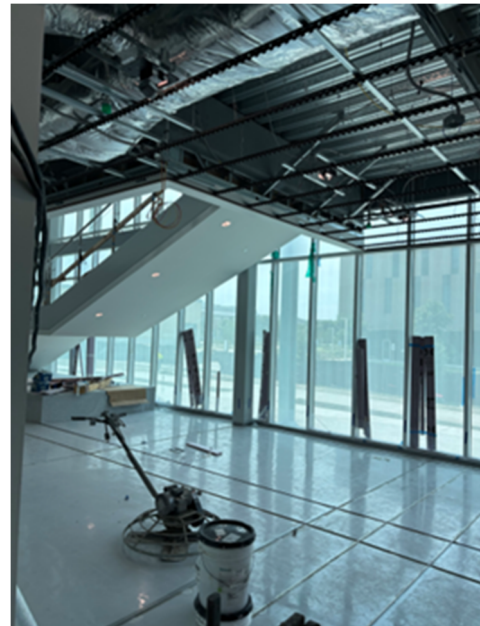
Level 1 – West Lobby Terrazzo Install
