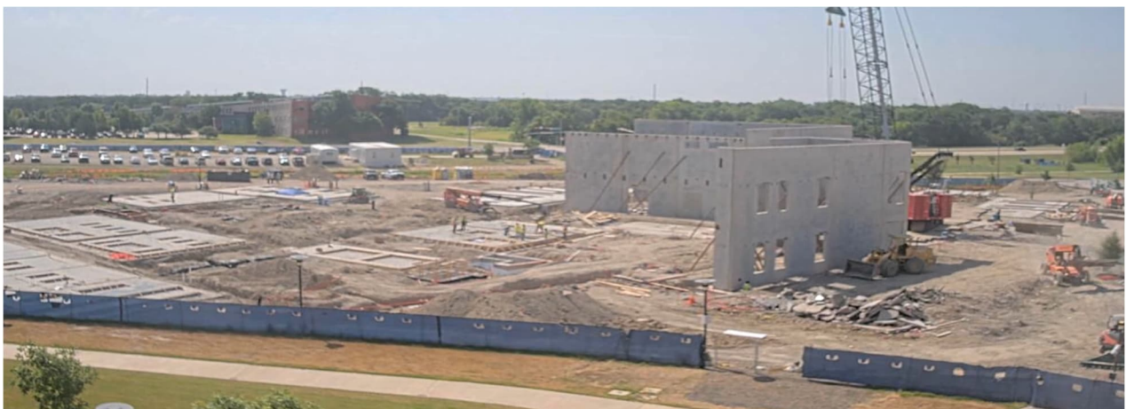
Tilt Wall Panel Erection
