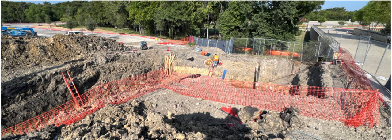
Excavation for Hydronic Piping
