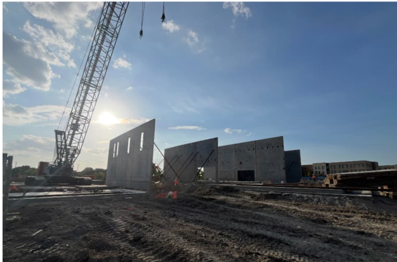
Tilt Wall Panel Erection
