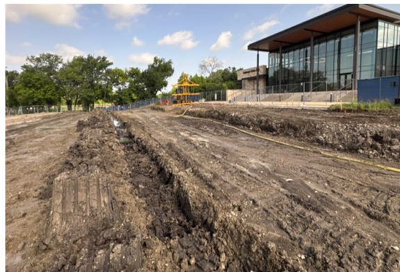
Grading for New Plaza
