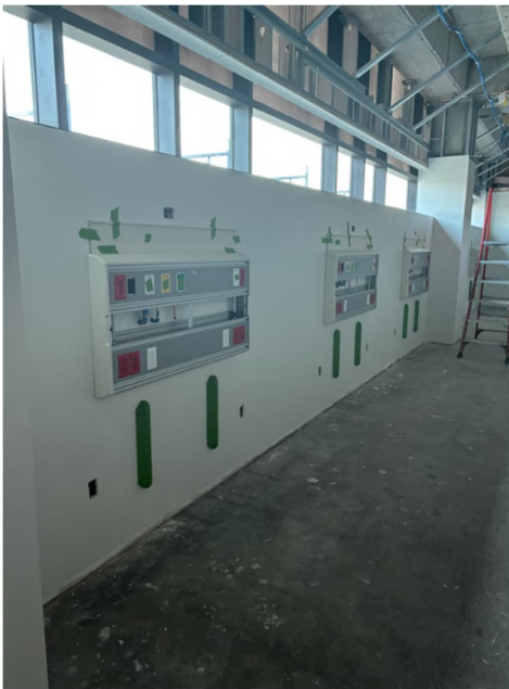
Nursing Skills South Wall
