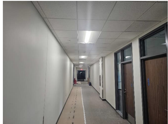
E Wing 1st Floor Hallway
