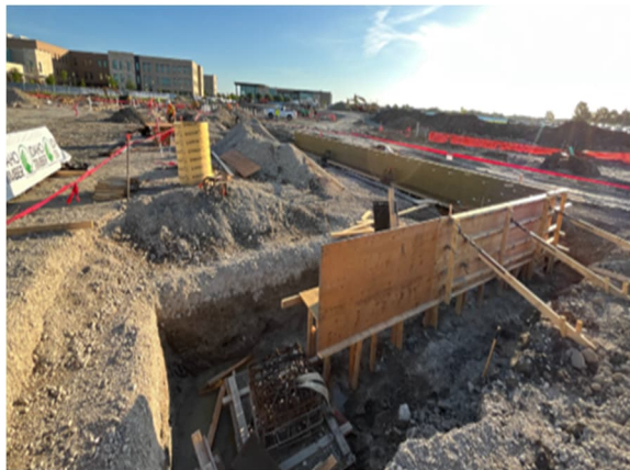
Forming Grade Beams
