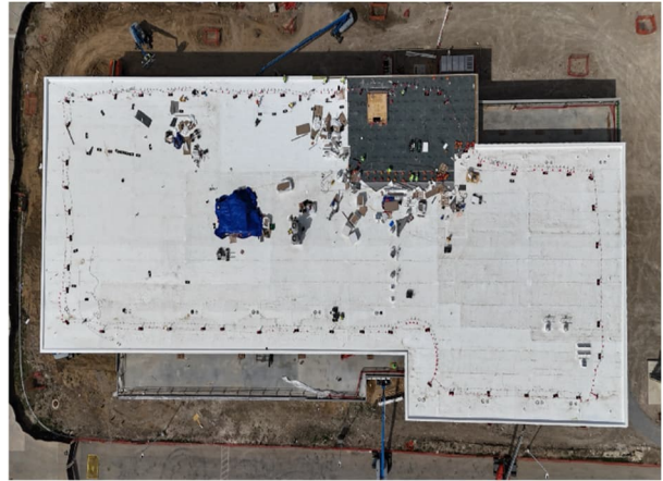
High Roof Nearing Final Membrane Roll-out
