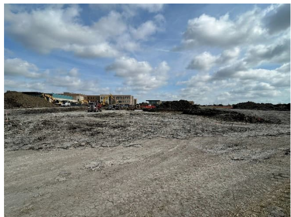
Site Excavation and Grading
