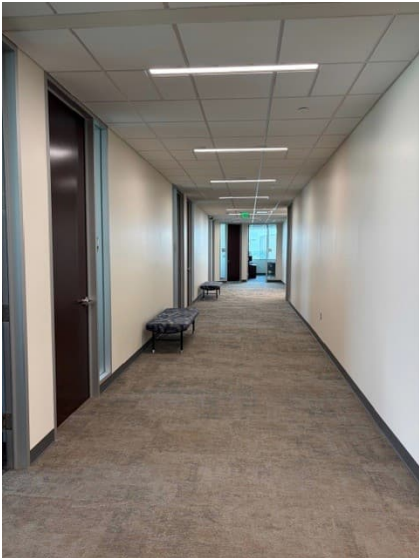
4 th Floor – Phase 3 New Offices
