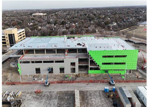
South Elevation – Sheathing and Waterproofing Installations
