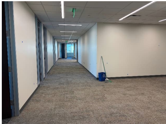
4th Floor – Phase 3 New Offices
