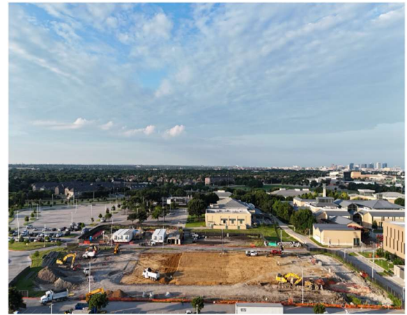
View Looking South
