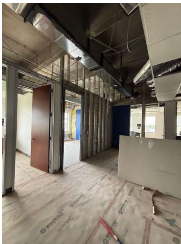
4th Floor – New office at IT area
