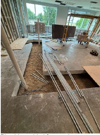
Plumbing added for new lounge area
