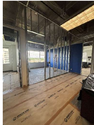
4th Floor – New office at IT area
