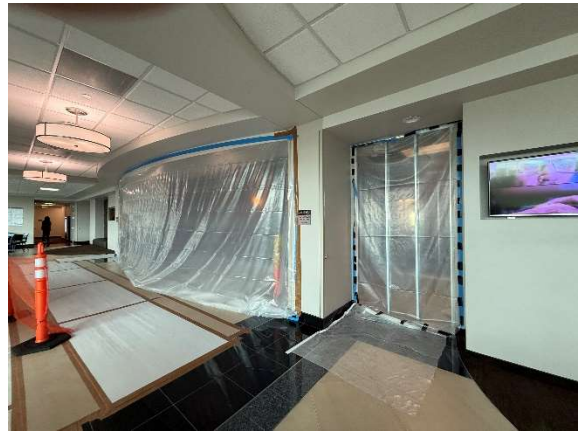
Second Floor Reception Area
