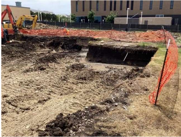
Excavation West End of Site
