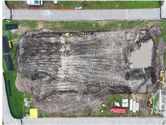
Overview of Site
