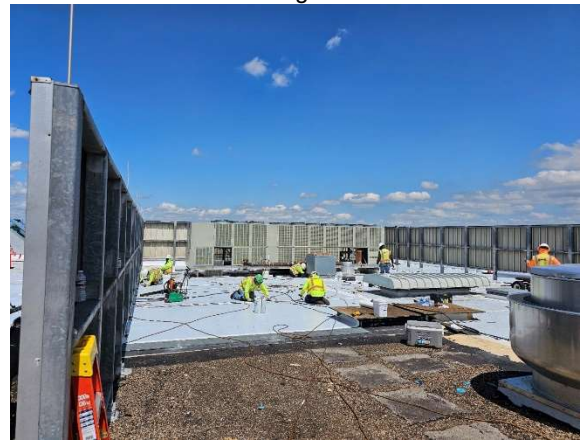
Roof Chiller Back in Place
