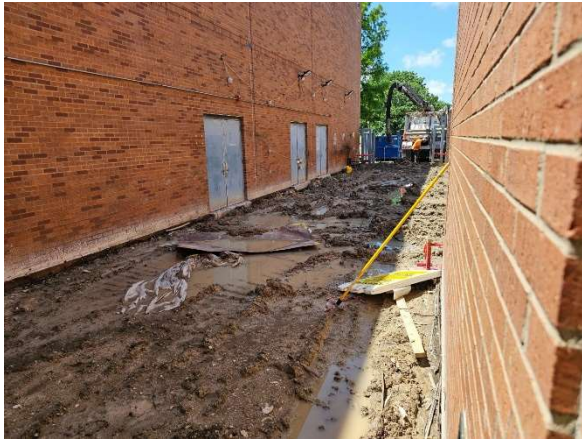
Fine Arts Courtyard Paving Demo Complete
