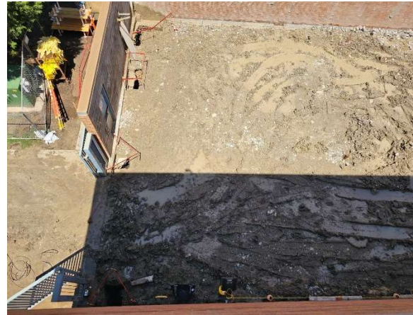
Fine Arts Courtyard Exploration Holes for Footing locations
