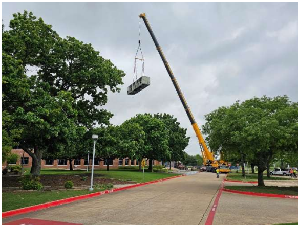
Roof Chiller Removed to Allow for Roof Work
