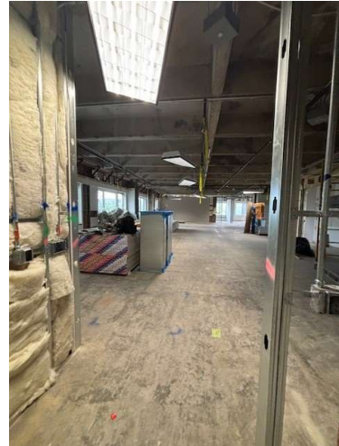
2nd Floor – Esthetician Lab, Insulation and One-sided Walls
