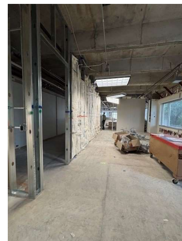
2nd Floor – Medical Massage Lab Storage, Insulation in Walls
