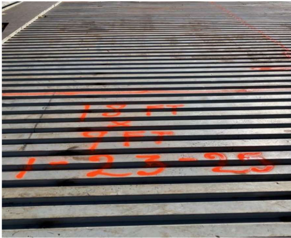
Existing Roof Metal Deck
