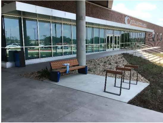
Seating in Front of North Building, NW View
