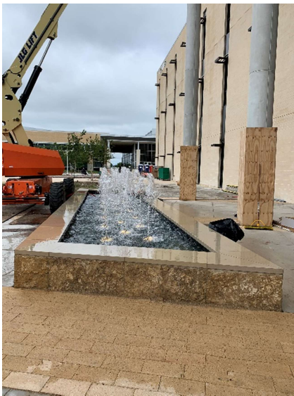
Water Feature Installed
