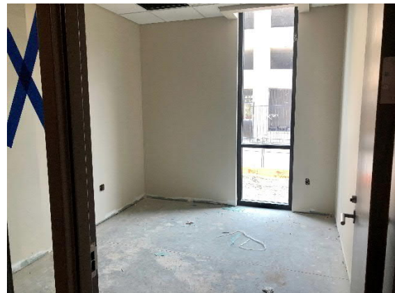
Faculty Office Space on 1 st Floor, NE End of Building
