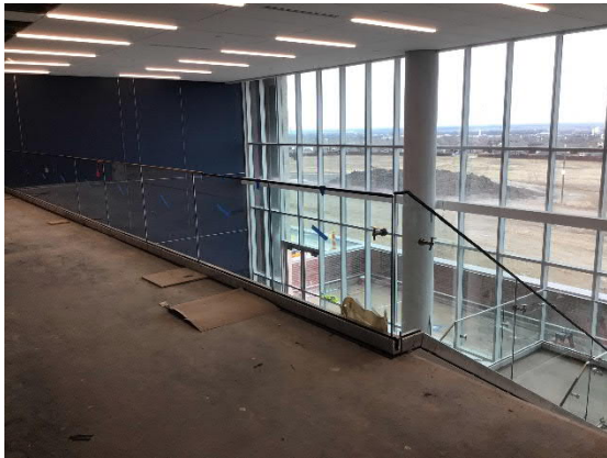
Glass Handrail Installed at Staircase
