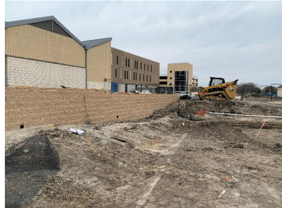
Retaining Wall, North of Alumni Hall
