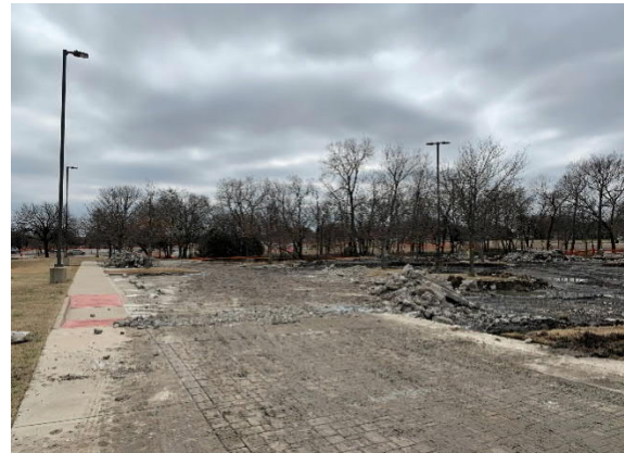
Demolition of Existing Paving at New Parking Lot
