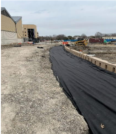
Prep for Concrete Pour at Retaining Wall
