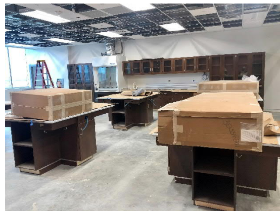
Lab on 2 nd Floor on South Building
