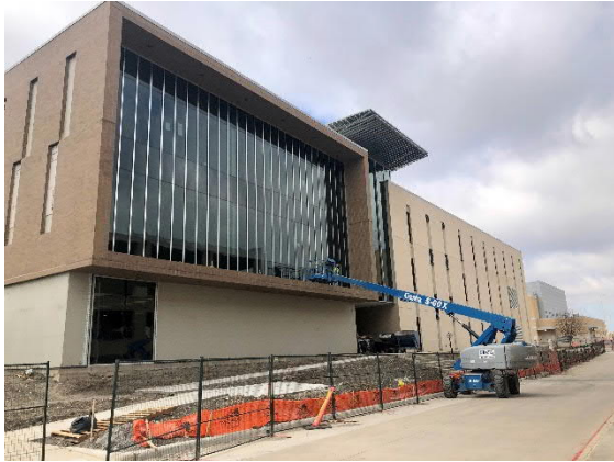
NE View of Building
