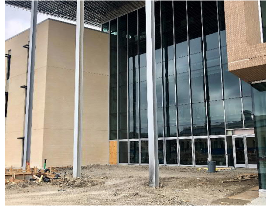
Main Entrance to Atrium
