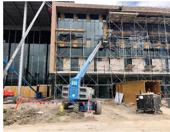
Glazing on South Façade of Area C
