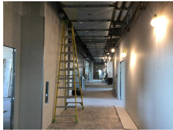
Second Floor Hall in North Building
