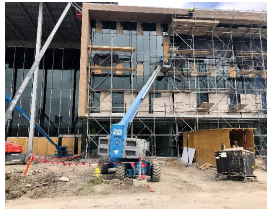
Glazing on South Façade of Area C
