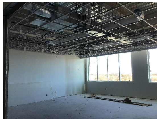
Second Floor Classroom Space in North Building
