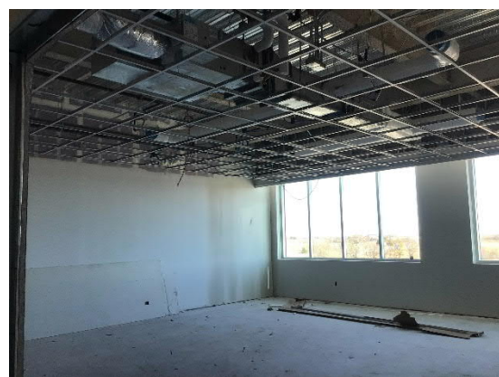
Second Floor Classroom Space in North Building
