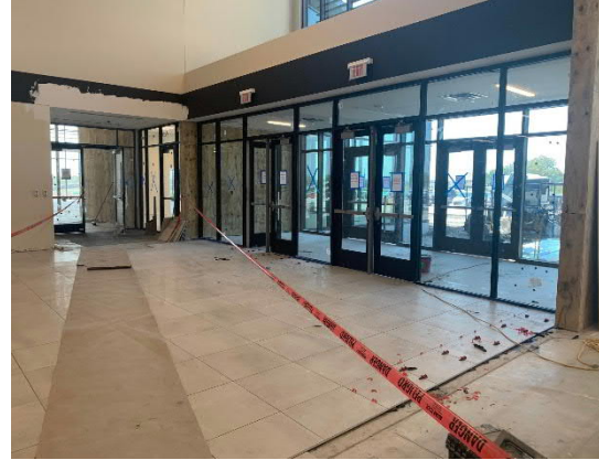
Floor Tile Installed at Lobby
