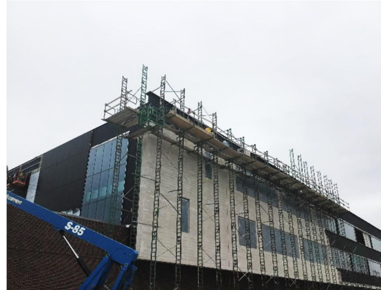
Block Work at East Elevation
