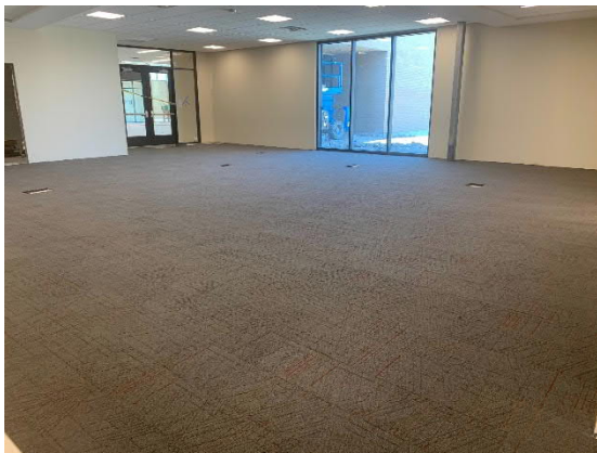
Carpet Installed at One-Stop Shop
