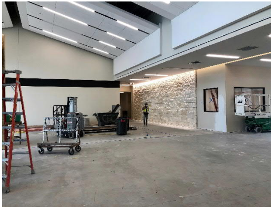
Commons Area at Main Entry
