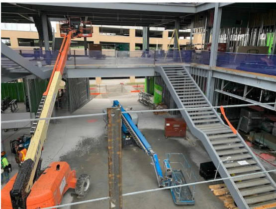
South View of Atrium from Level 2 Bridge
