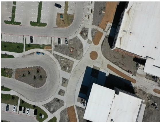
North View Aerial of Parking and Sidewalks
