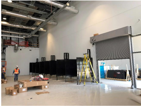
Welding Booth Installation at Trade Bar B
