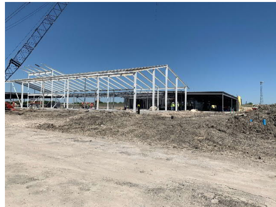
Southwest View of Library
