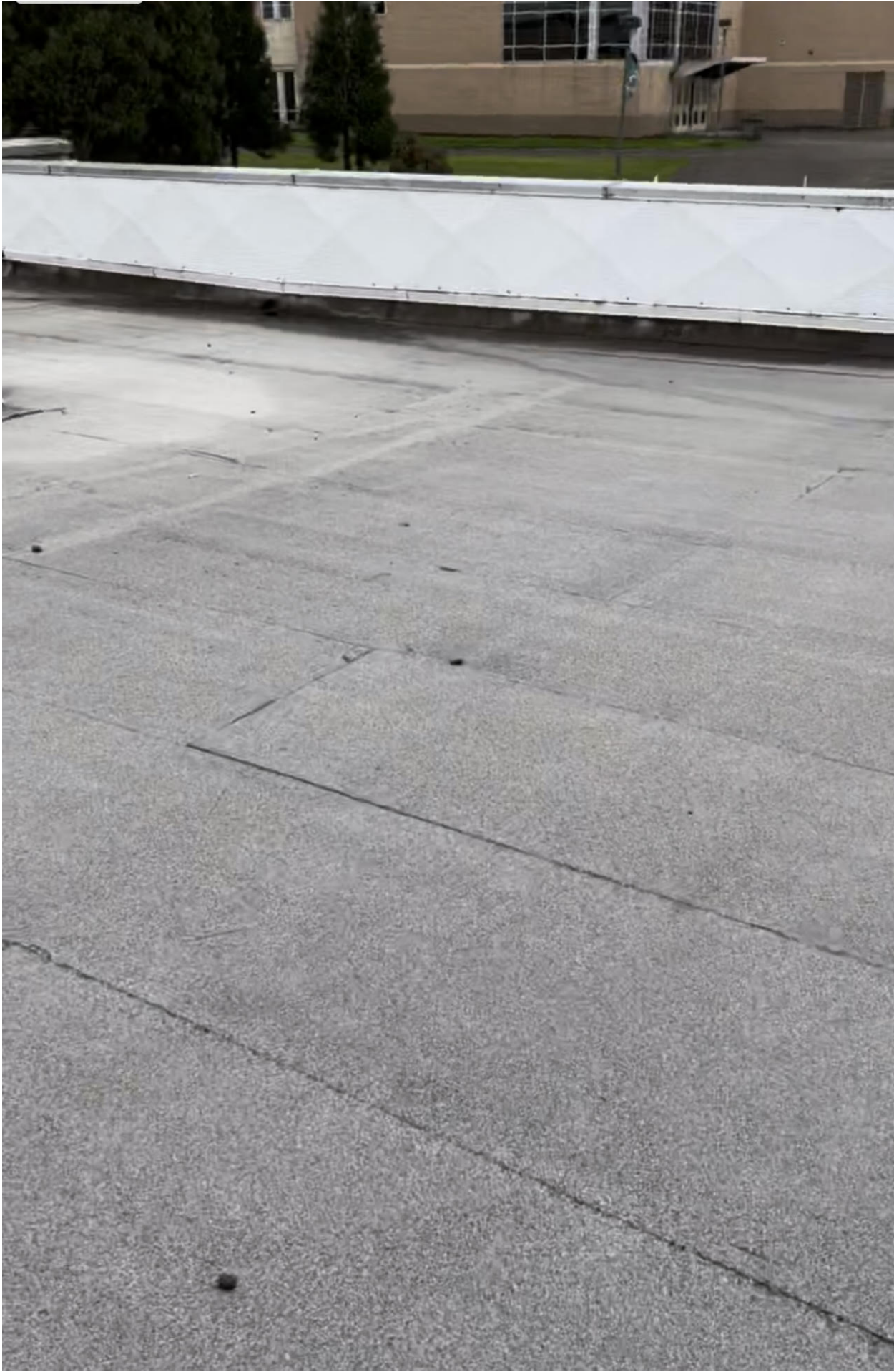
High School roof section 2H
