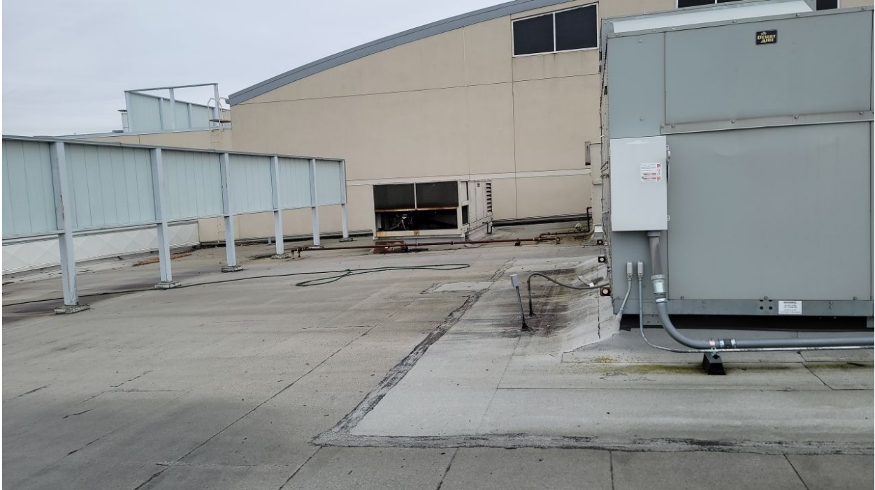
High School roof section 2H
