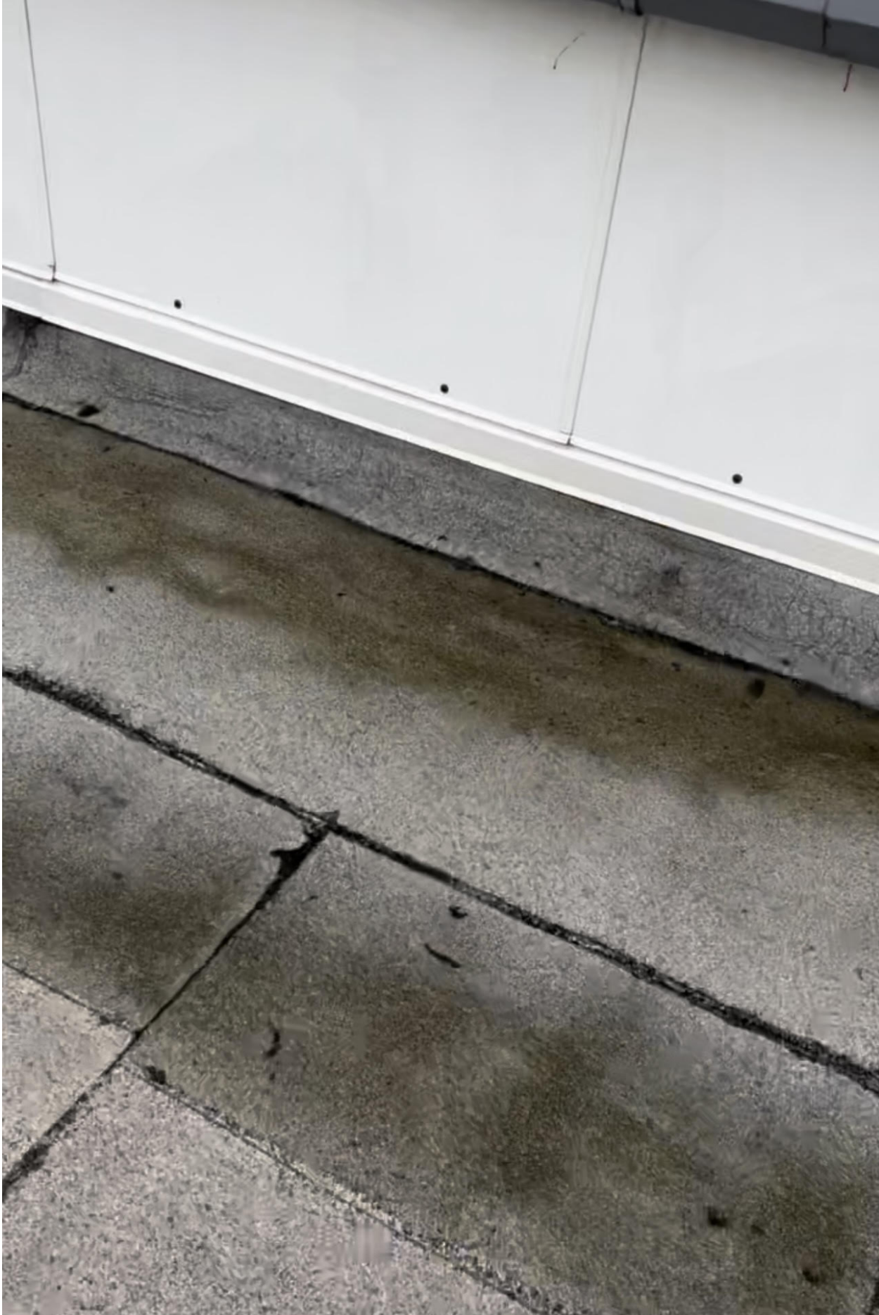
High School roof section 2H
