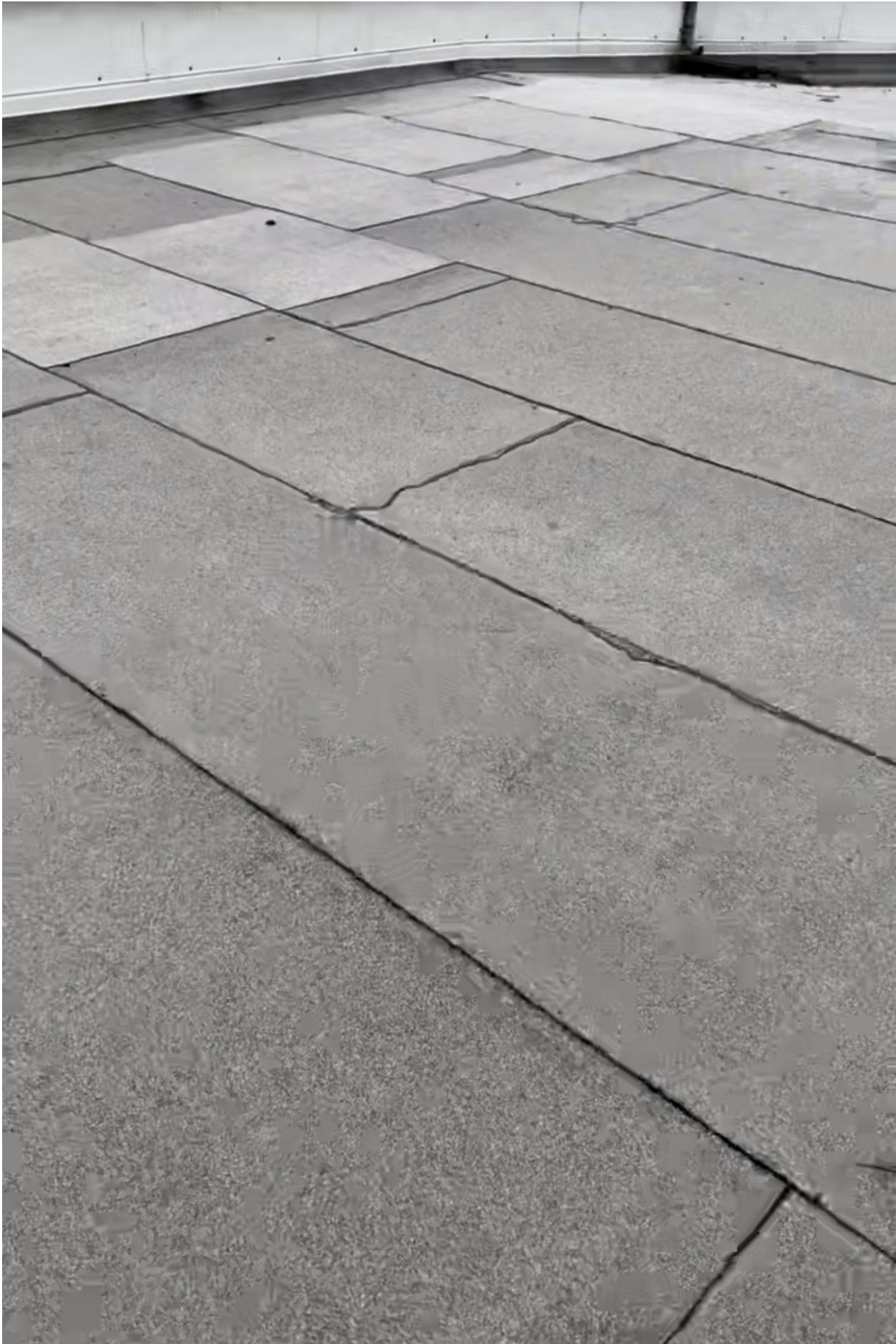
High School roof section 2H
