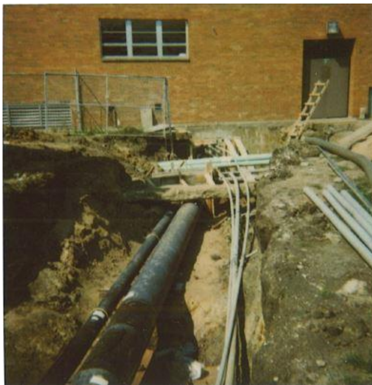
Picture 2 (GHS Steam Lines August 2000 – Looking toward HS)
