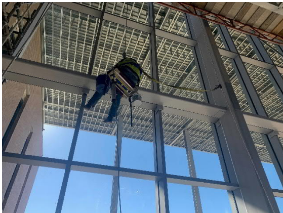
South Curtain Wall
