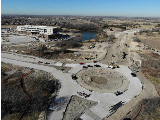
Roadway at West Entrance of Campus
