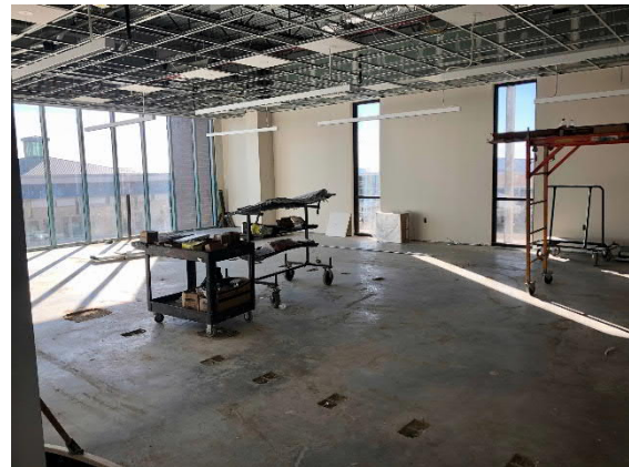
Rack Room on 3 rd Floor, South end of Building
