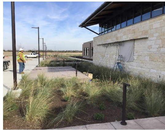
Signage Install at Main Entrance to Building
