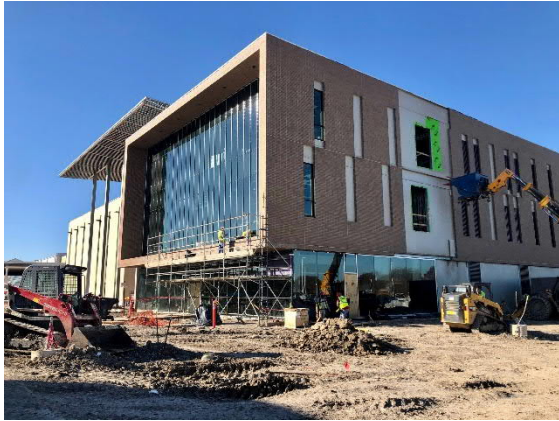
SE View of Building
