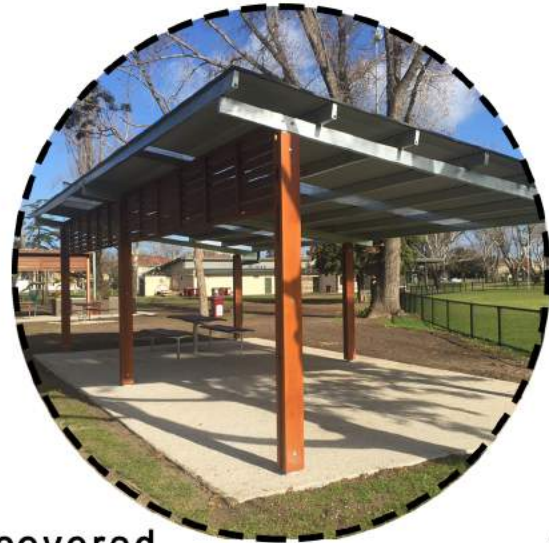
covered outdoor classroom
