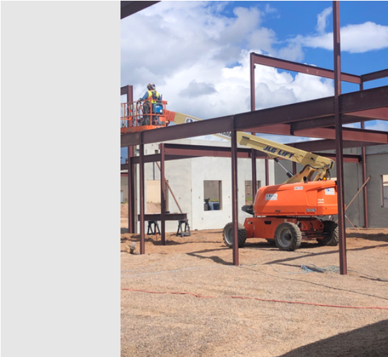
Description DSC Steel Erection
