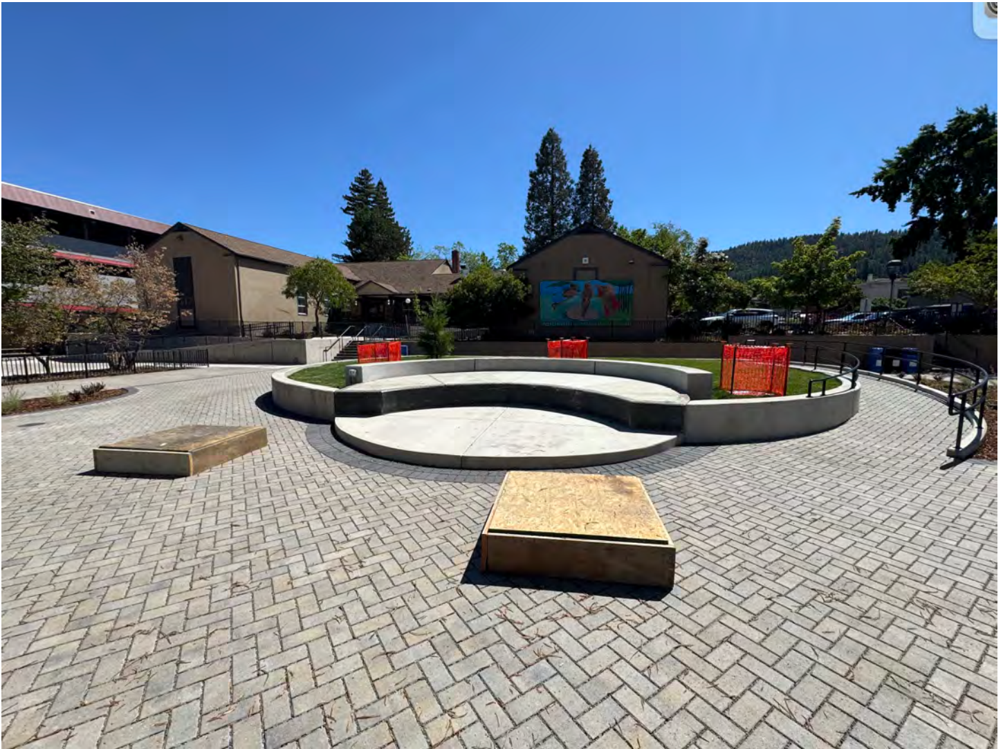
South Facing View of the Quad Renovations
