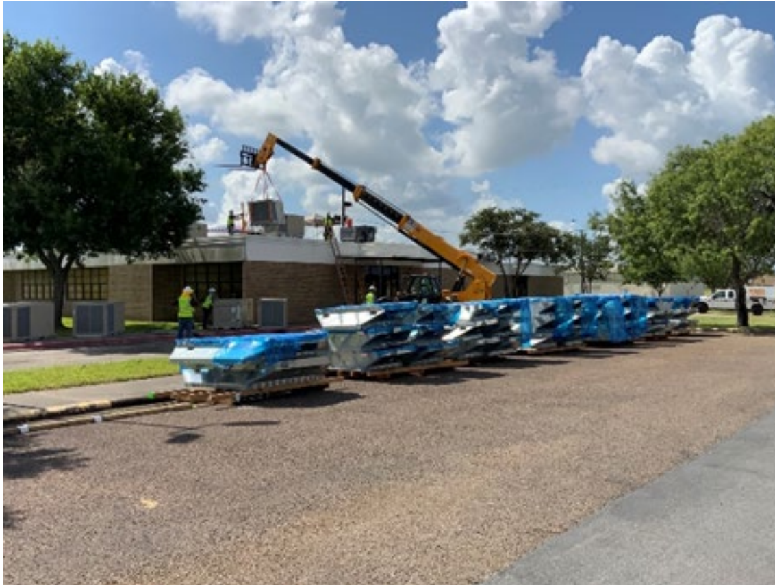
Installation at Gonzalez Elementary
