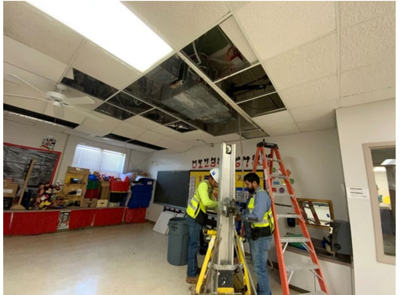
Repairs at Aiken Elementary
