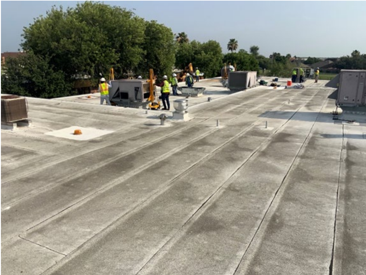
Installation of Yturria Elementary
