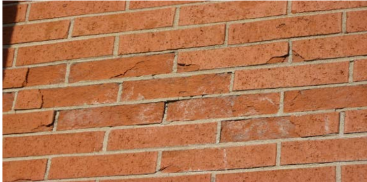
Spalling brick.
