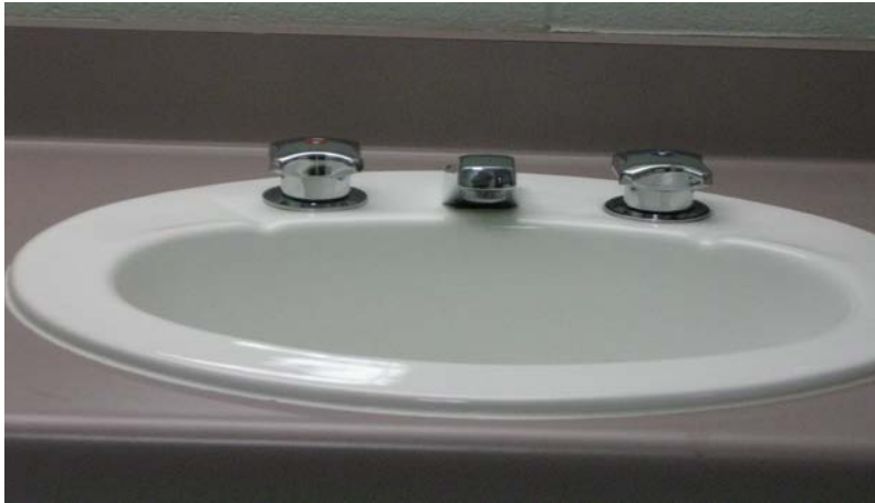
Replace fixtures with touchless fixtures.
