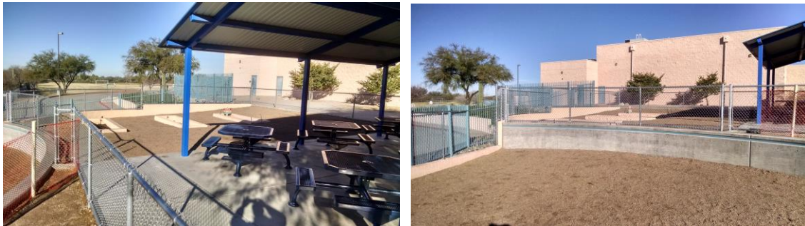
Courtyard Playground Improvements
