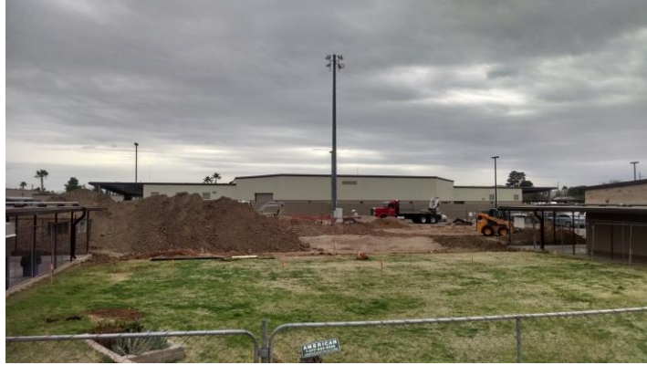
Over Excavation of Professional Development Building Pad
