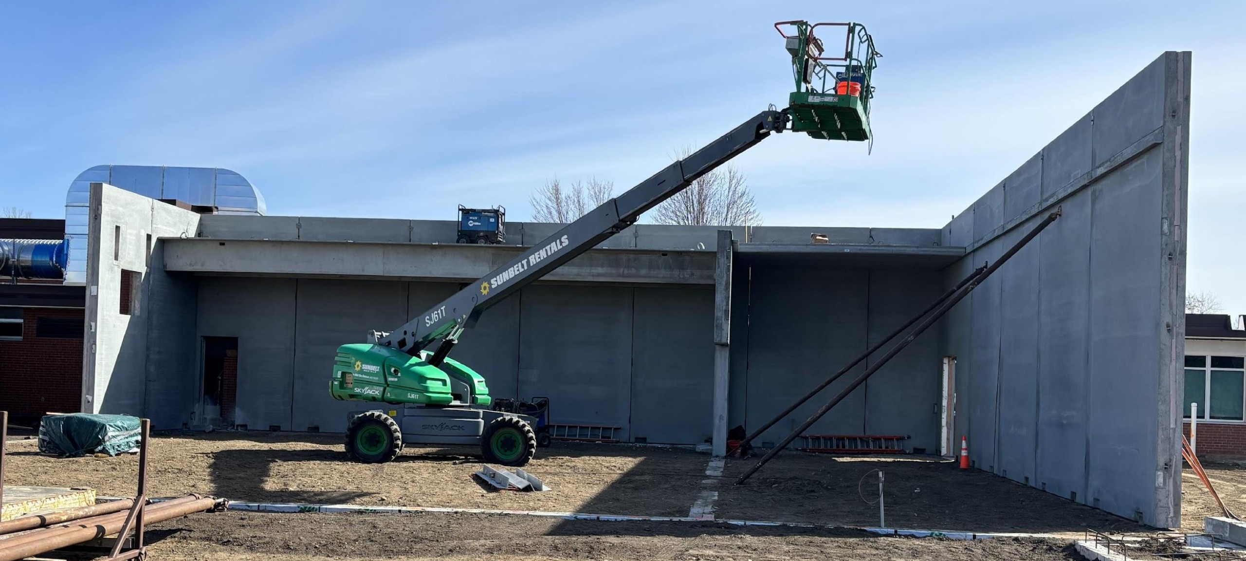
SLP Aquila Elementary – Flex Space Precast
