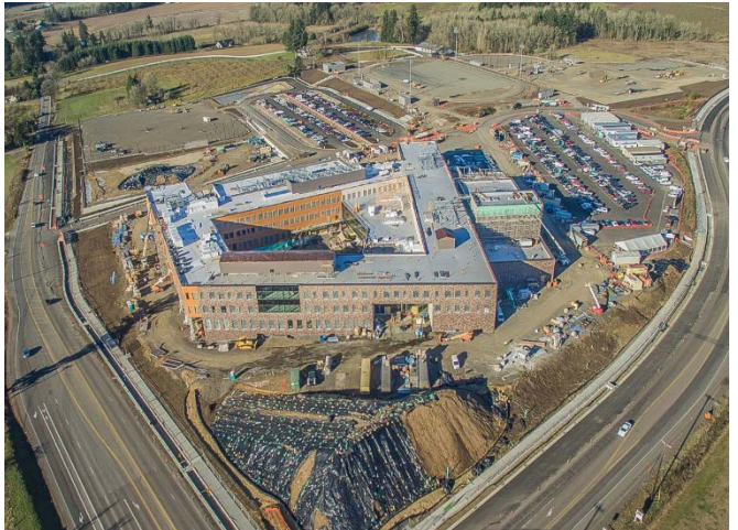
Site Aerial - looking west
