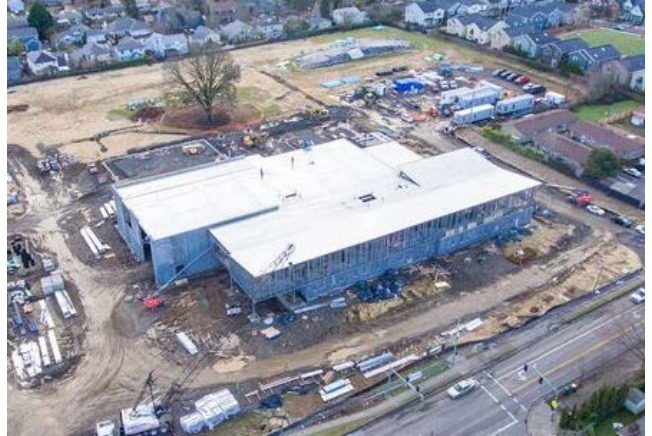
Site view – looking southwest
