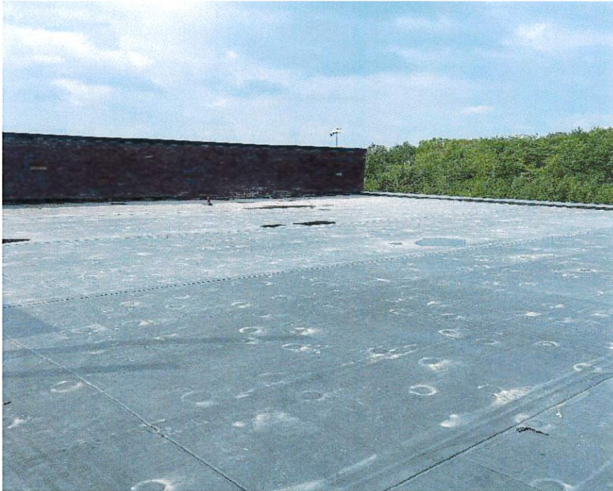
Brick removal area 1
