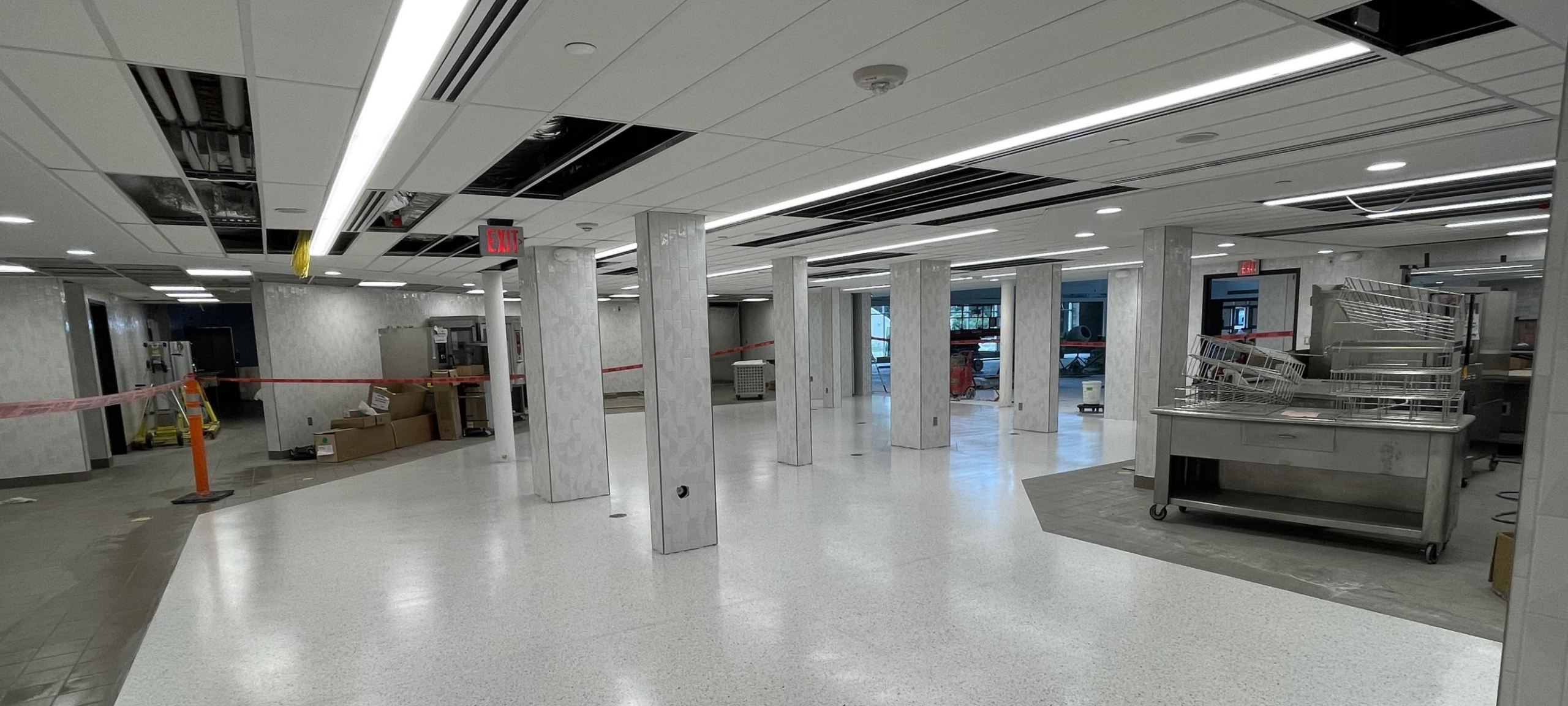
SLP High School – Cafeteria Kitchen
