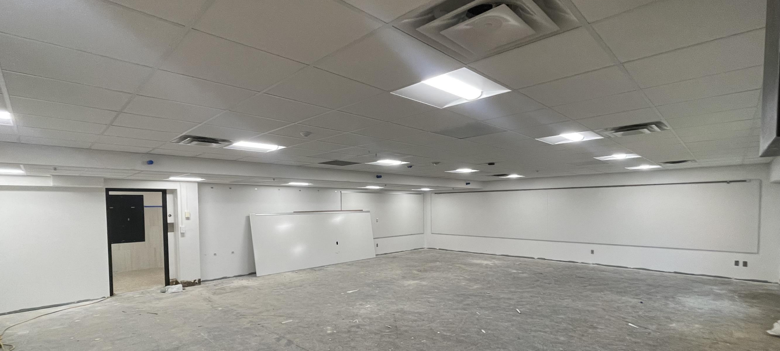
SLP HS Classroom Renovations Phase 2
