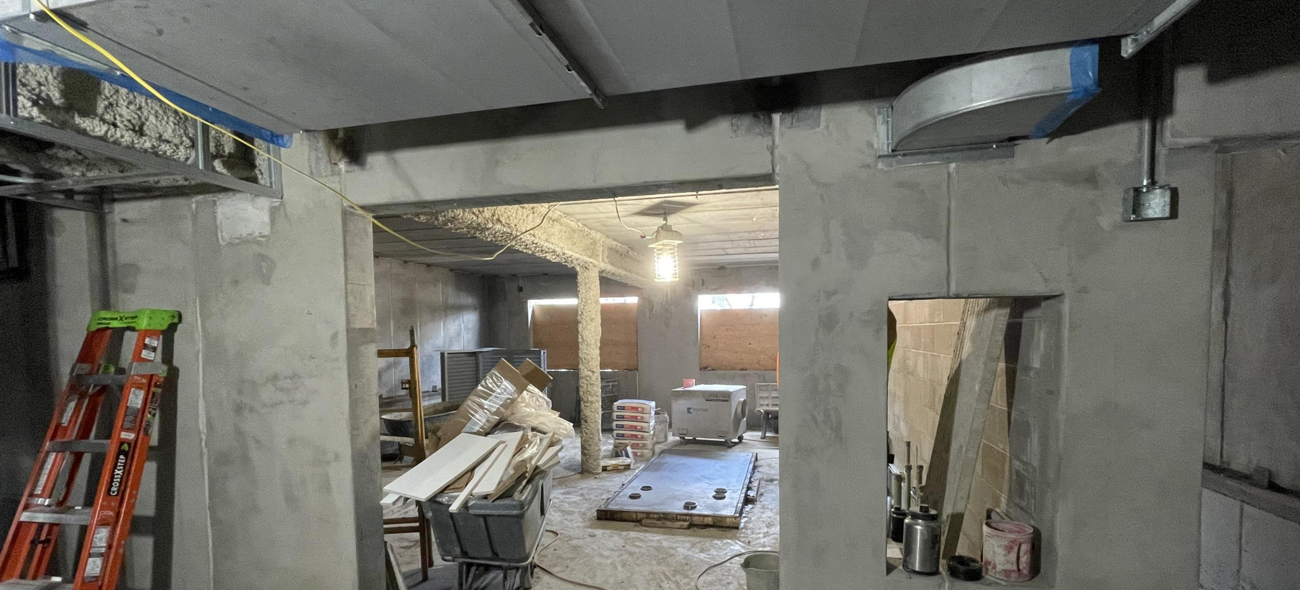
SLP High School – Storm Shelter
