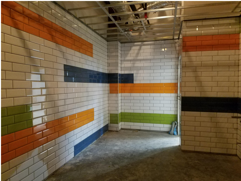
Tile work at Student Restroom.
