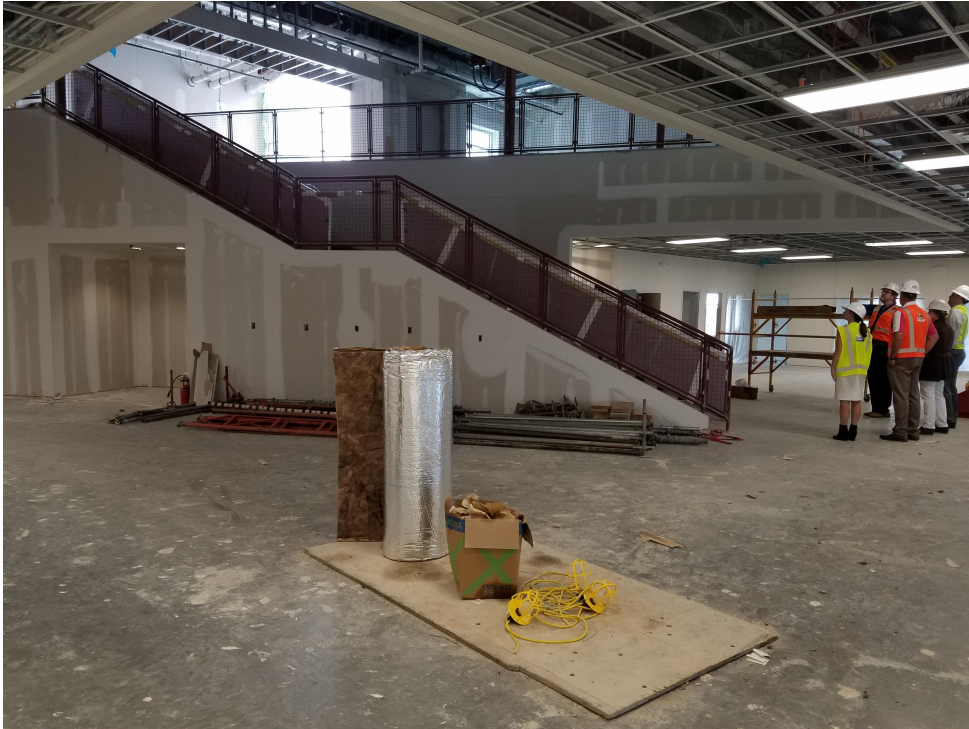
Area D Classroom Learning Stair.
