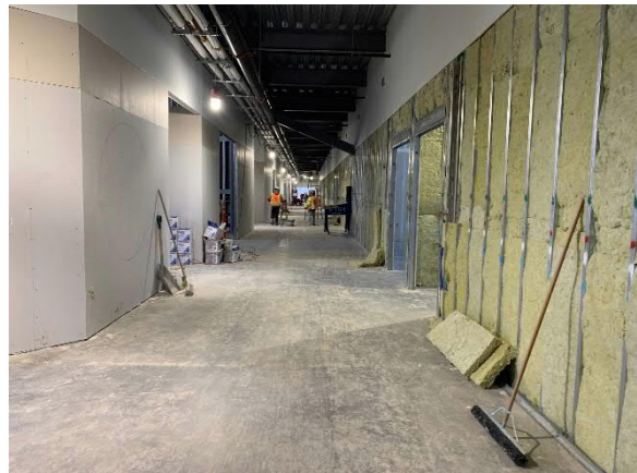
Insulation Installed at Trade Bar C
