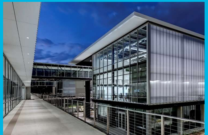
Exterior Walkways Between Academic Building and Trade Buildings
