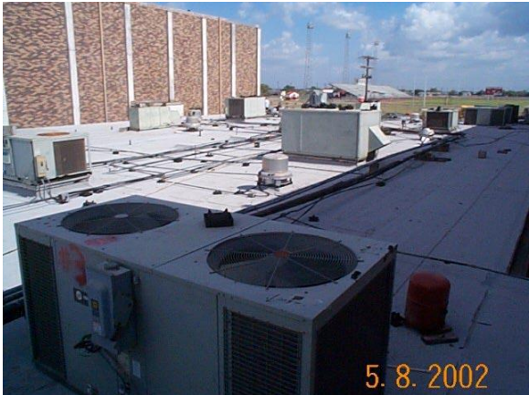
roof @ weight room
