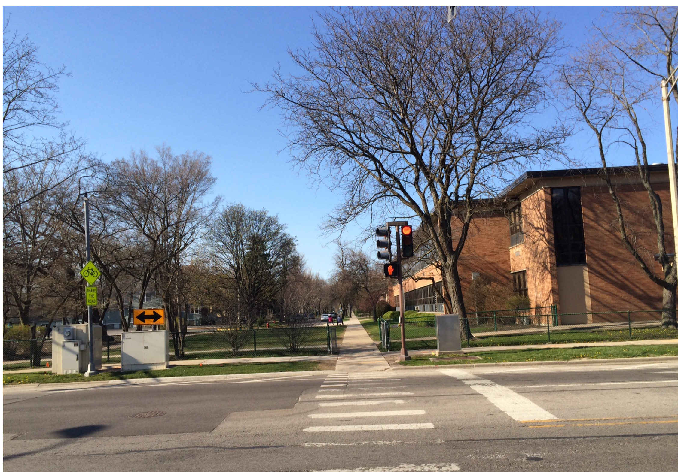
PHOTO LOOKING NORTH FROM CHICAGO AVE. SHOWING THE CONTINUITY OF WALK WAY AT THE FRONT OF THE BUILDING
